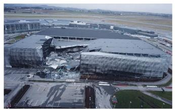
Figure 13: Stavanger airport carpark collapse after the fire. Reproduced from [60]. © Nordic Unmanned.
