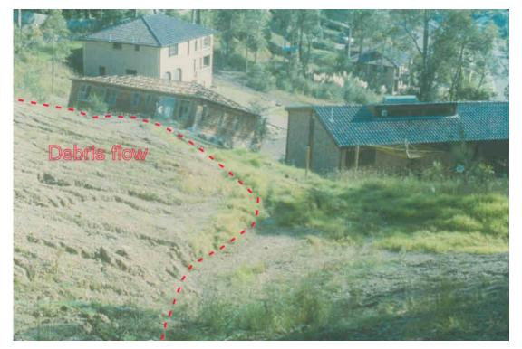
Figure 4 - Impact of fast moving landslide (Photograph courtesy of Max Ervin)
