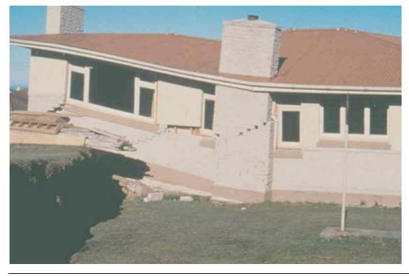
Figure 5 – House damage following a landslide (Photograph courtesy of Max Ervin)
